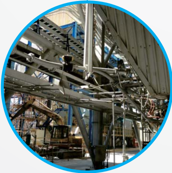
>> Pneumatic Conveying System
